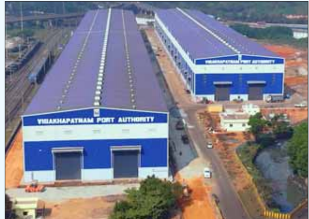
Covered storage sheds in Port area
