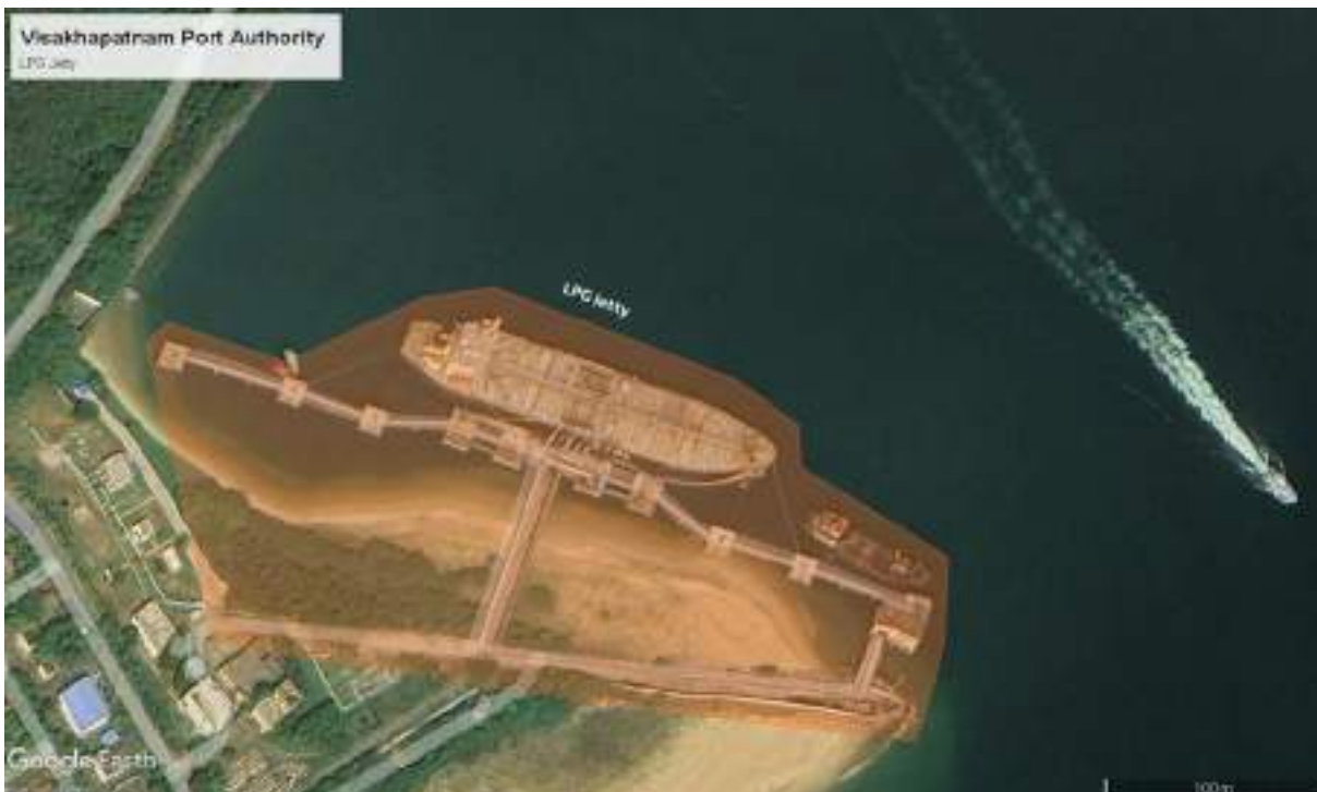
Figure 5-10 LPG Jetty of VPA
