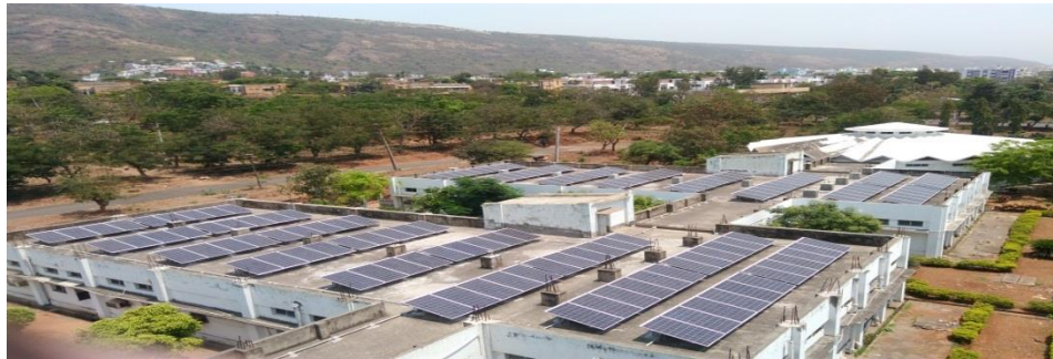
Solar Panel installed at GJH
